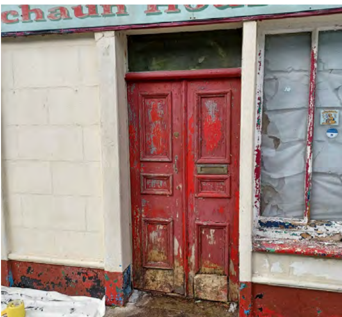
Tulla House Before
