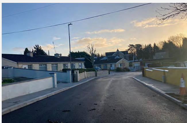
Beechwood Lawn, Bodyke – Upgrade December 2021.
