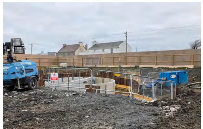
Construction of storm storage tank at John P Holland Park, Liscannor.
