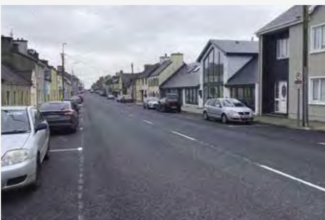
Miltown Malbay Church Street road improvement works.
