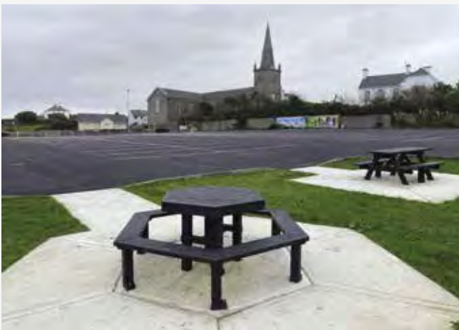
Miltown Malbay Church Car Park works, supported by The Ireland Funds.
