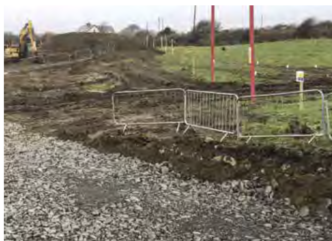
WWTP excavations for new structures.
