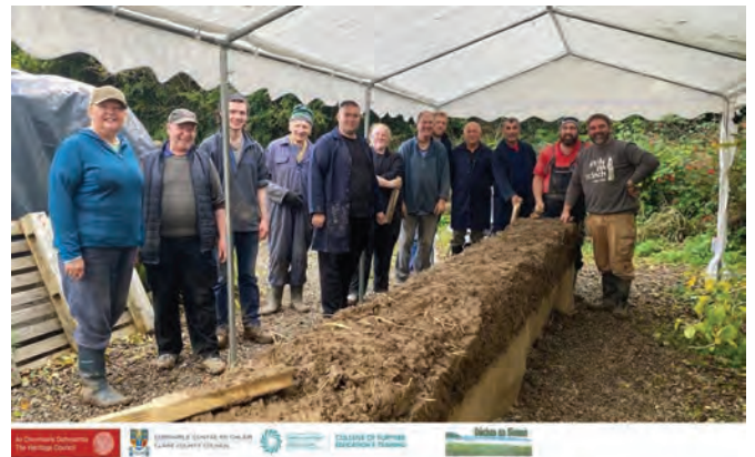
Training in vernacular forms of construction at Hastings Farmhouse.
