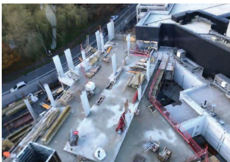
Progress photograph from October 2022
