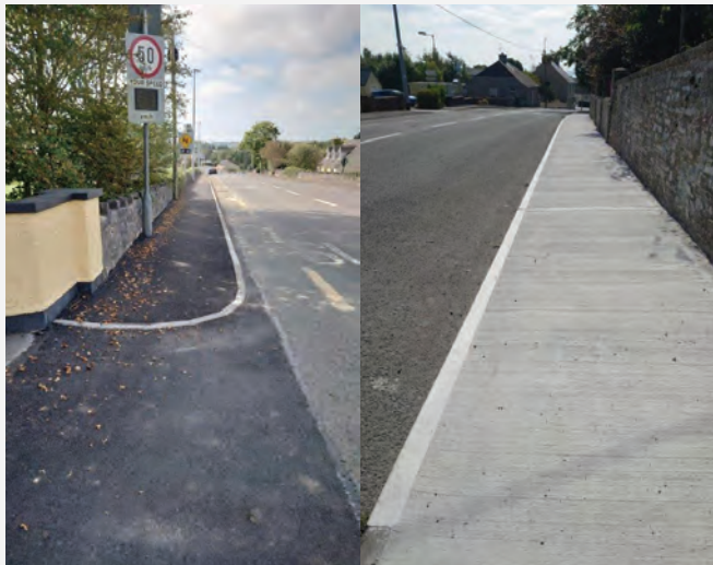
Above left: Active Travel footpath on Ennis Road, Killadysert, on approach to school and town. Above right: Active Travel footpaths in Killadysert Village R473.
