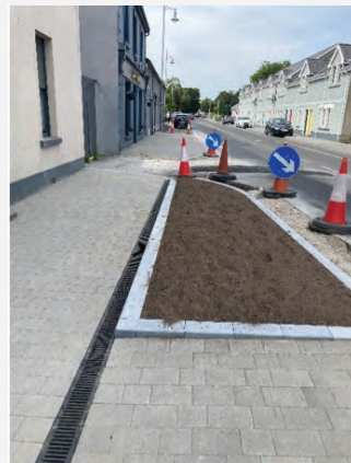
Public realm works in Clarecastle.
