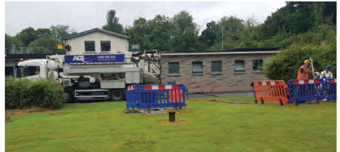
Cleaning Clearwater Tank At Castlelake WTP.
