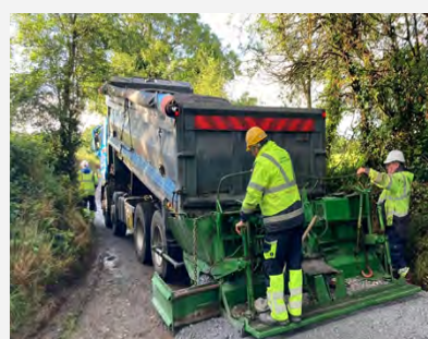
Killaloe MD crew restoring roads in July.
