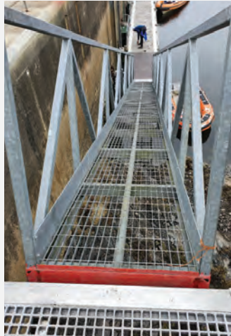
Doonmore Pier. Ramped access platform now in place.
