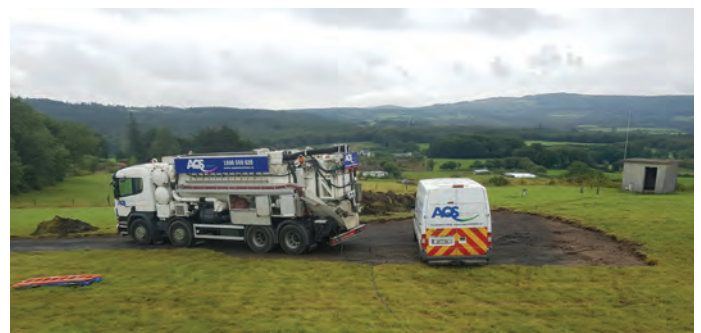
Cleaning Moygalla Reservoir.
