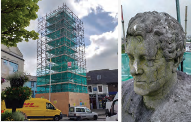
Conservation works on the Daniel O'Connell Monument.
