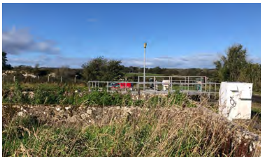
Existing Kilfenora WWTP
