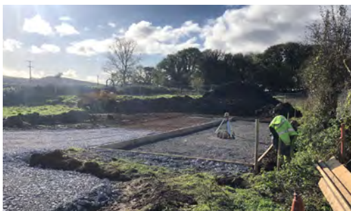
Kilfenora WWTP temporary works
