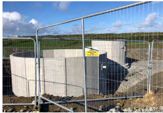
Liscannor WWTP tanks under construction
