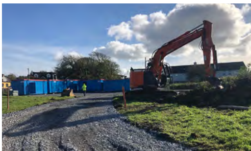
Kilfenora WWTP temporary site compound and fencing
