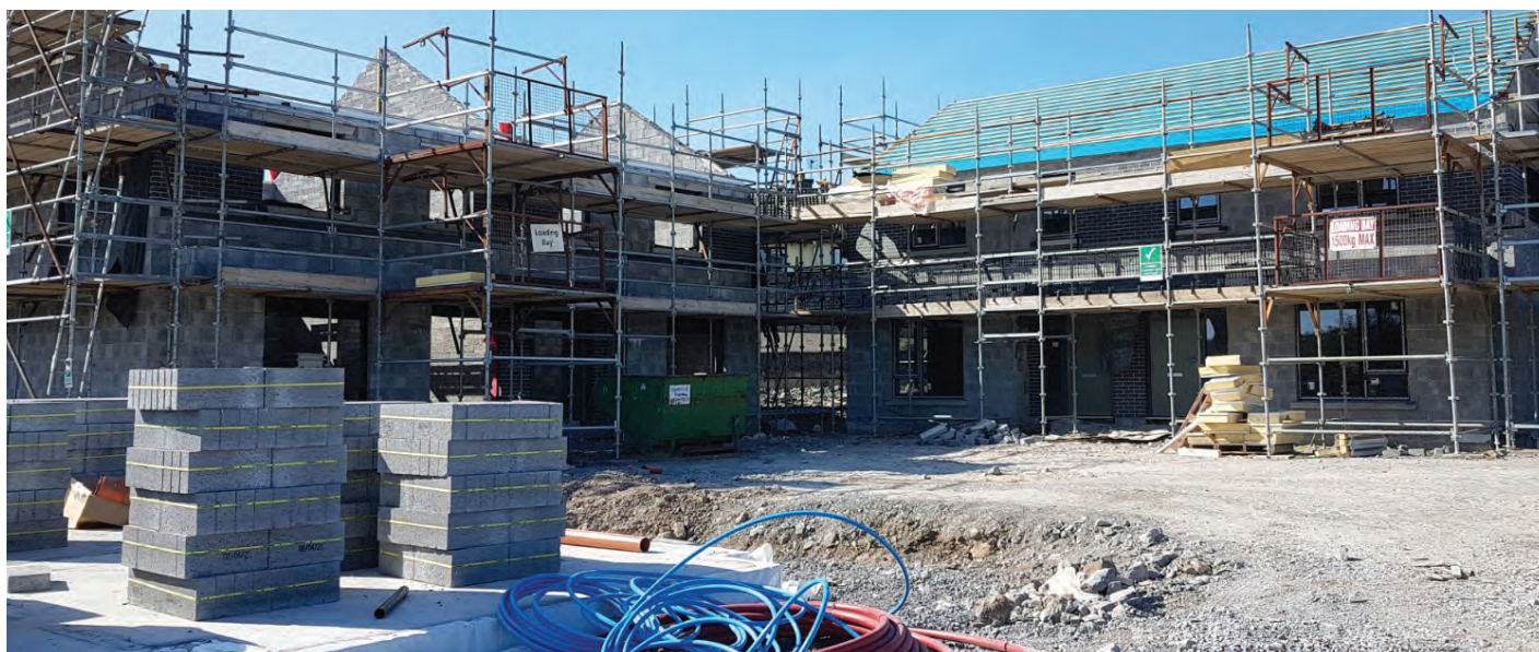
Ashline social housing development.
