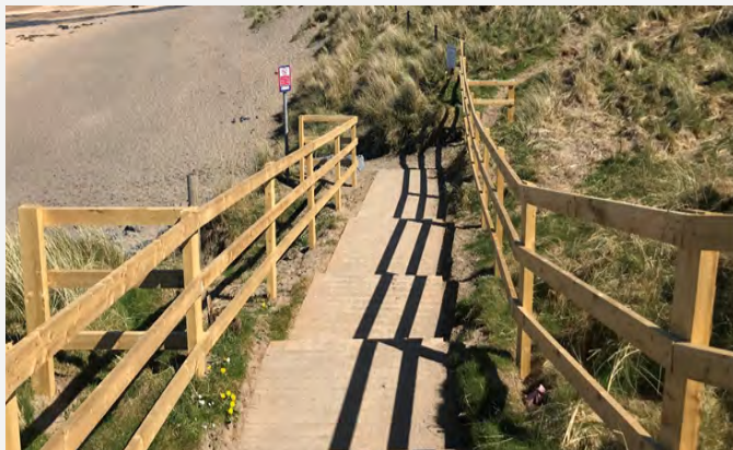
Fanore beach works.
