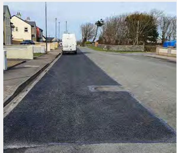
Localised Planing & Resurfacing Works Recently completed at Dún na Mara, Doonbeg.
