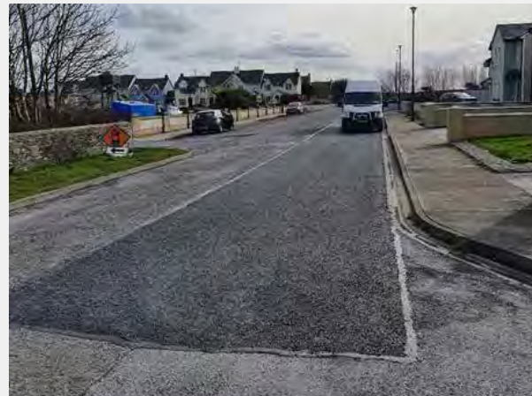
Localised Planing & Resurfacing Works Recently completed at Dún na Mara, Doonbeg.
