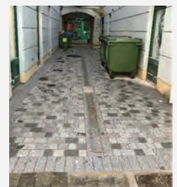
Completed paving to River Lane.
