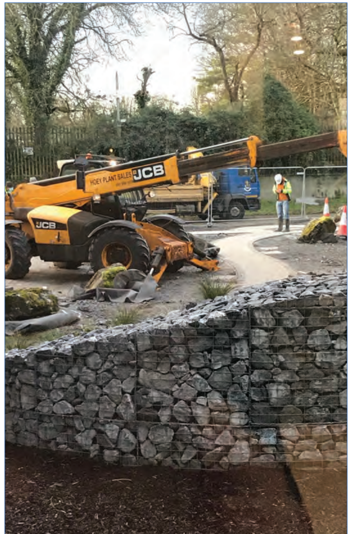
Works progressing on the reflective garden.
