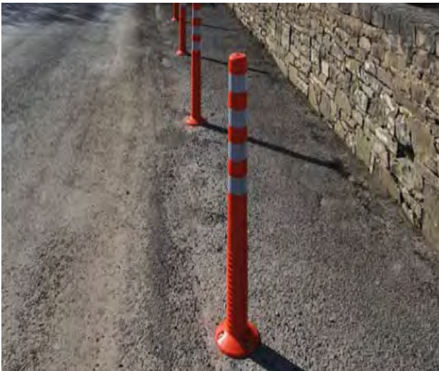
Annagh National School. Recently installed traffic bollards.
