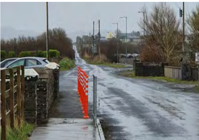
Annagh National School. Recently installed traffic bollards.
