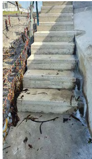
Pedestrian access steps. Viewed from slipway.
