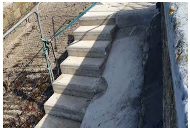
Pedestrian access steps. Viewed from roadside footpath.
