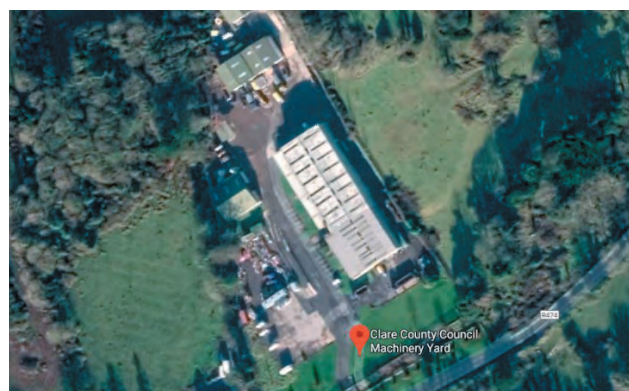
Beechpark Machinery Yard Buildings
