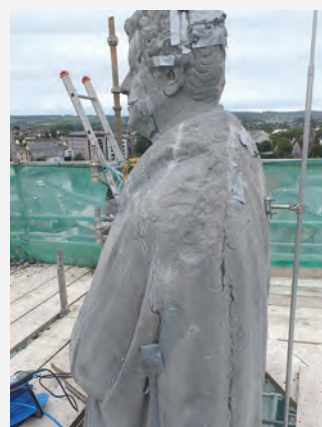
The sealing of the cracks has just commenced (above left). The holes in the face are being left as found.
