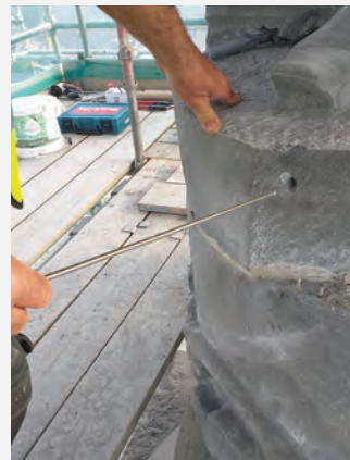
The sealing of the cracks has just commenced (above left). The holes in the face are being left as found.
