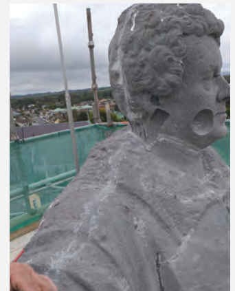
The sealing of the cracks has just commenced (above left). The holes in the face are being left as found.
