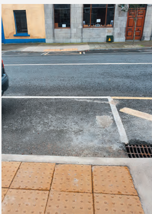
Kilrush Moore Street - Pedestrian Crossing - Dropped Kerbs & Tactile Paving
