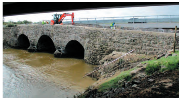
Latoon Bridge works - during repair.
