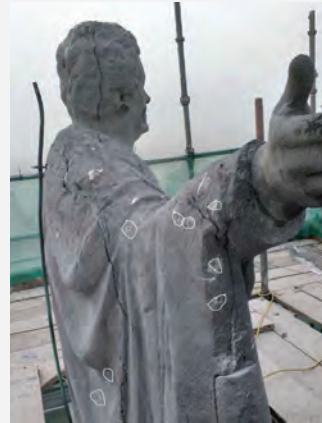
It is difficult to see where the drilling and stitching has taken place, as the filler is the same finish as the stone.
