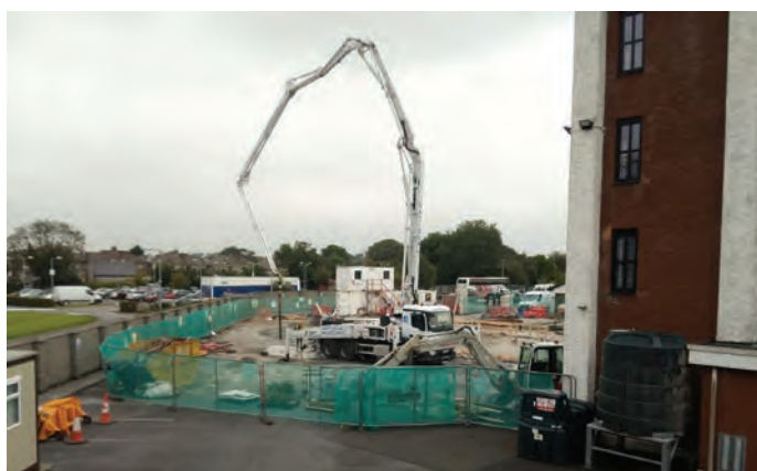
Ennis Fire Station redevelopment works are progressing.
