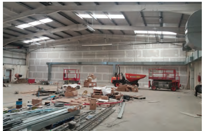
Civil Defence garage area.
