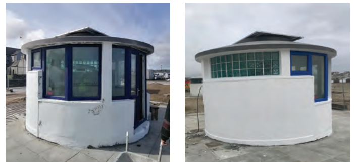
Kilkee beach hut refurbishments.
