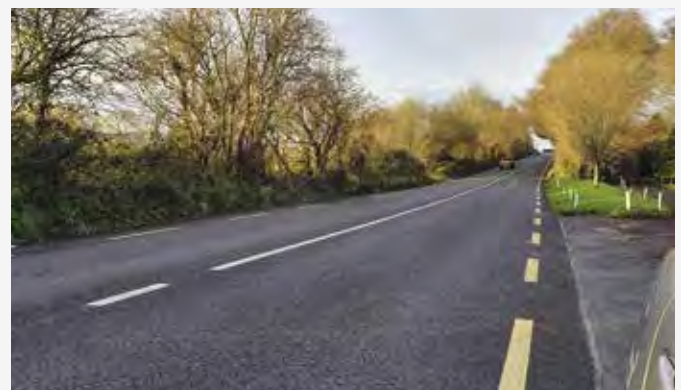
Pavement Overlay Works at Rosmadda.
