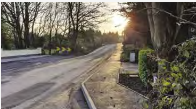
New footpath and road drainage installed in Meelick village.
